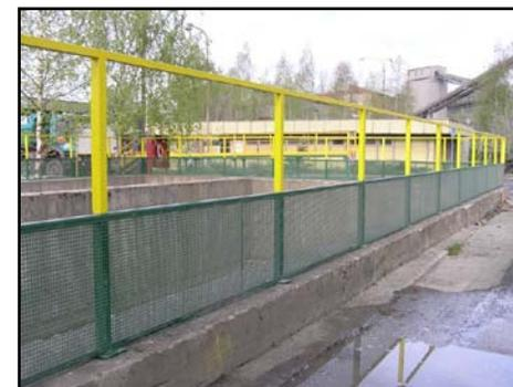
A technical barrier around the water pool, with vertical walls to protect small animals from potential falls into the pool.
