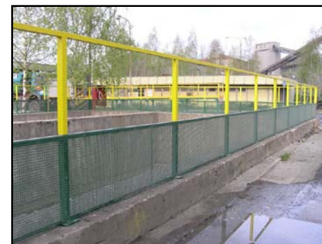
A technical barrier around the water pool, with vertical walls to protect small animals from potential falls into the pool. Děpoltovice quarry, 2006
